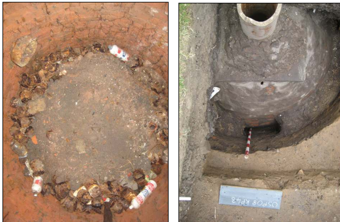
Fig 3: The brick structure
